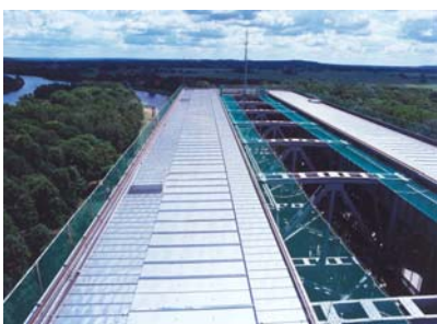
Ship lift, Niederfinow
